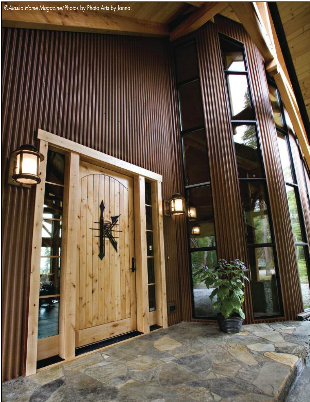
THIS RESIDENCE IN SOLDOTNA, ALASKA, USED ASC BUILDING PRODUCTS' COUNTRY RUSTIC CORRUGATED METAL SIDING TO PROVIDE A NICE LOOK AND SEAMLESS FINISH.
