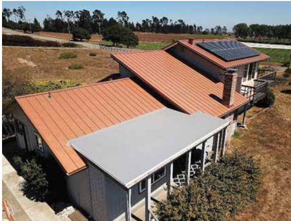
Skyline roofing featuring solar panels
