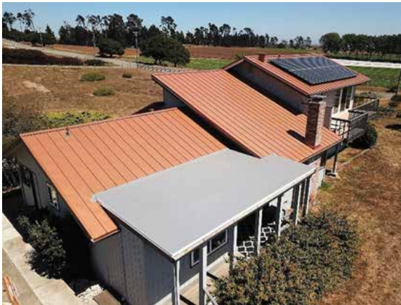
Skyline roofing featuring solar panels
