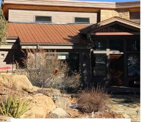
**Safe.** Metal roofs will not ignite or support combustion during a wildfire or lightning strike.
